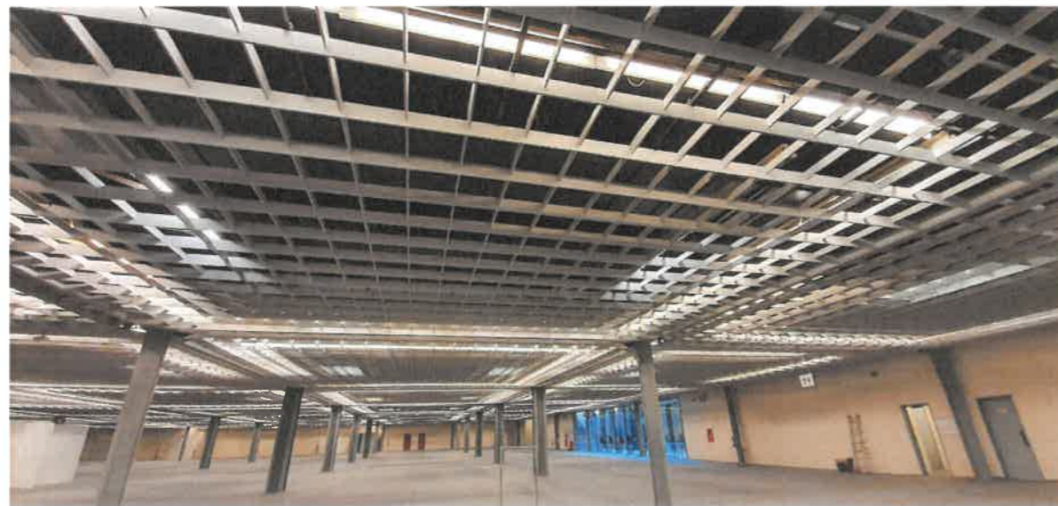
ADMITTED APPENDAGES TO CROSSED STRUCTURE ONLY, OVER THE FALSE CEILING (grating approximately 1.00 x 1.20 m)
